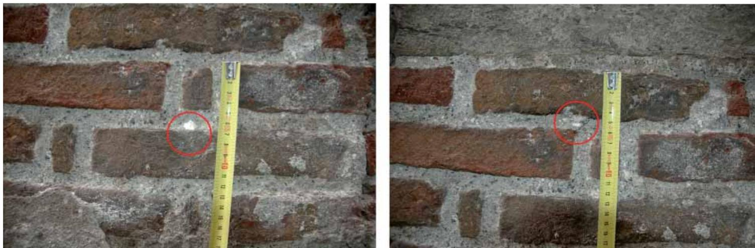
Fig.1 - Details of the sampling points of the lump n. 7 (left hand side) and 6 (right hand side)
