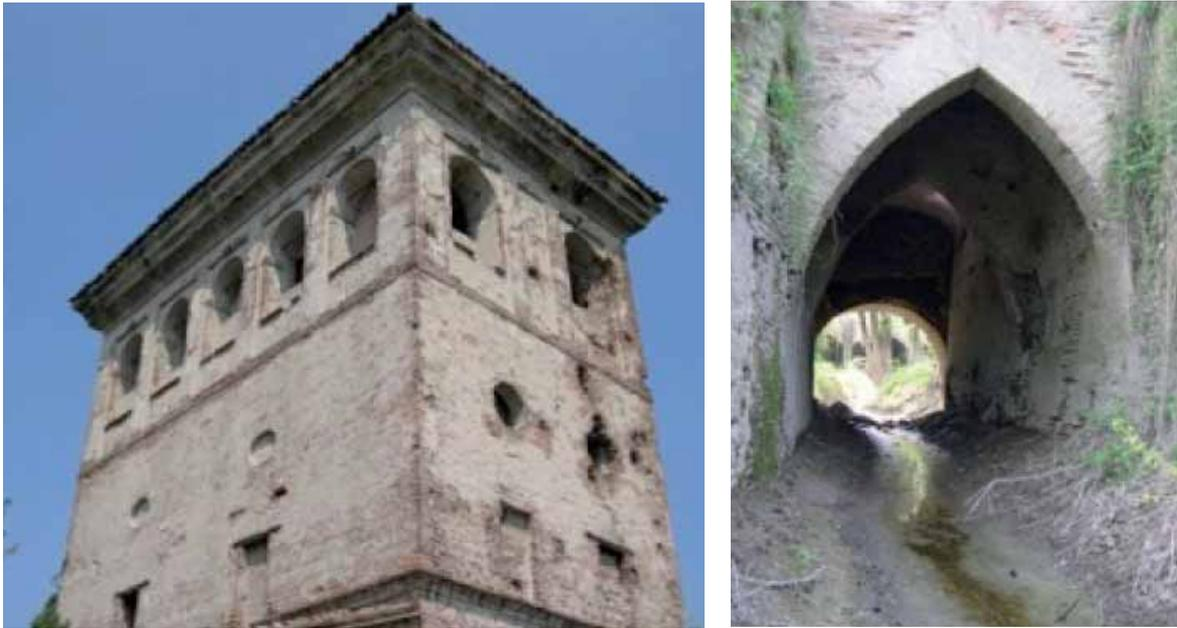
Fig.3 - On the left, south view of the Tower of Waters; the great ogival vault on the Galasso canal, which constitutes the foundation of the tower
